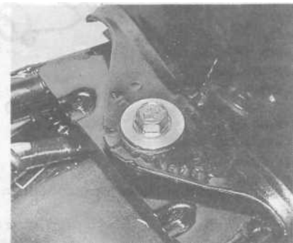
11.1 Petrol tank rear mounting is secured by a single bolt
